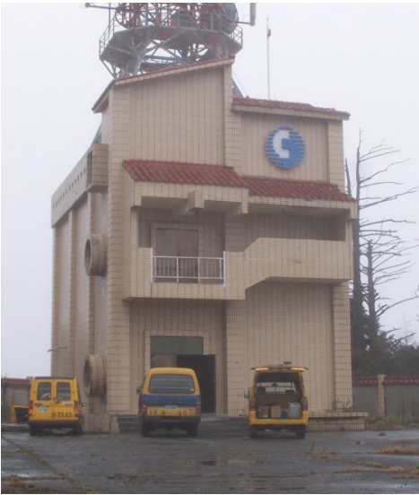
Figure 13. Chunghwa Telecom's central office
