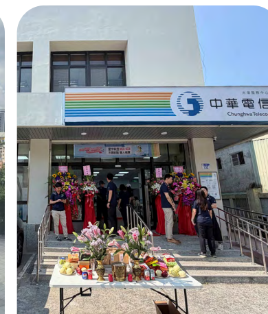
Figure 13. Chunghwa Telecom's service center and office building
