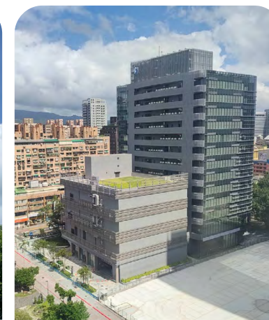
Figure 12. Chunghwa Telecom's telecom facilities
