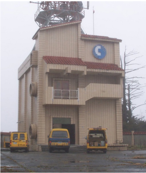
Figure 13. Chunghwa Telecom's central office
