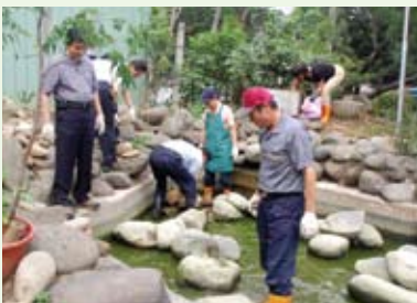
An ecological pond was built at an open space.
